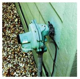
FIGURE 1 Bonding clamp attached to a gas regulator.
